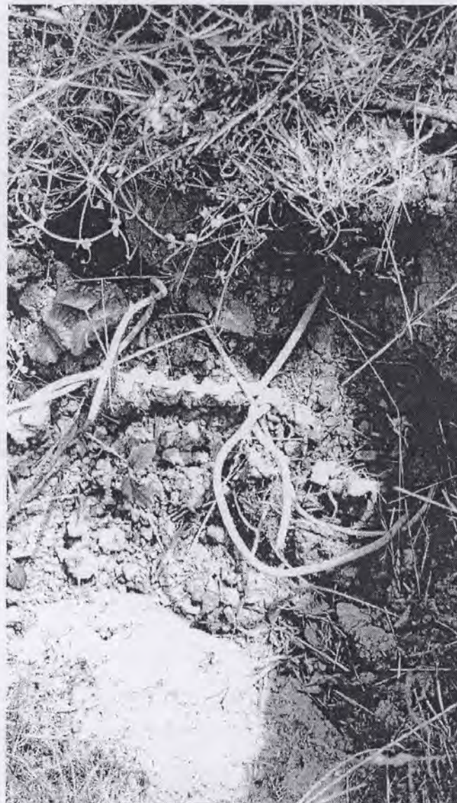
PTB/Fig. 32: #4 ground wires
