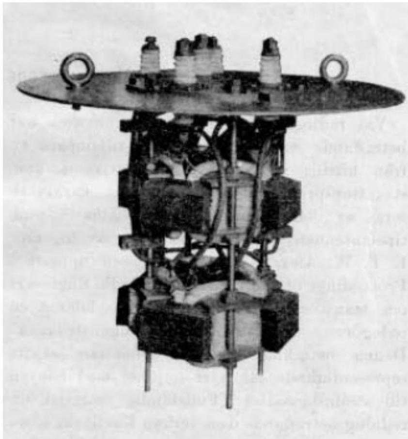
Fig. 3. The magnetic amplifier in the transmitter in Grimeton
