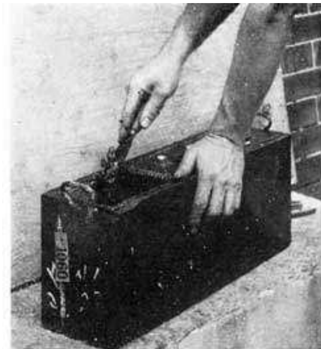
Fig. 200. Removing Compound from Top of Jar
