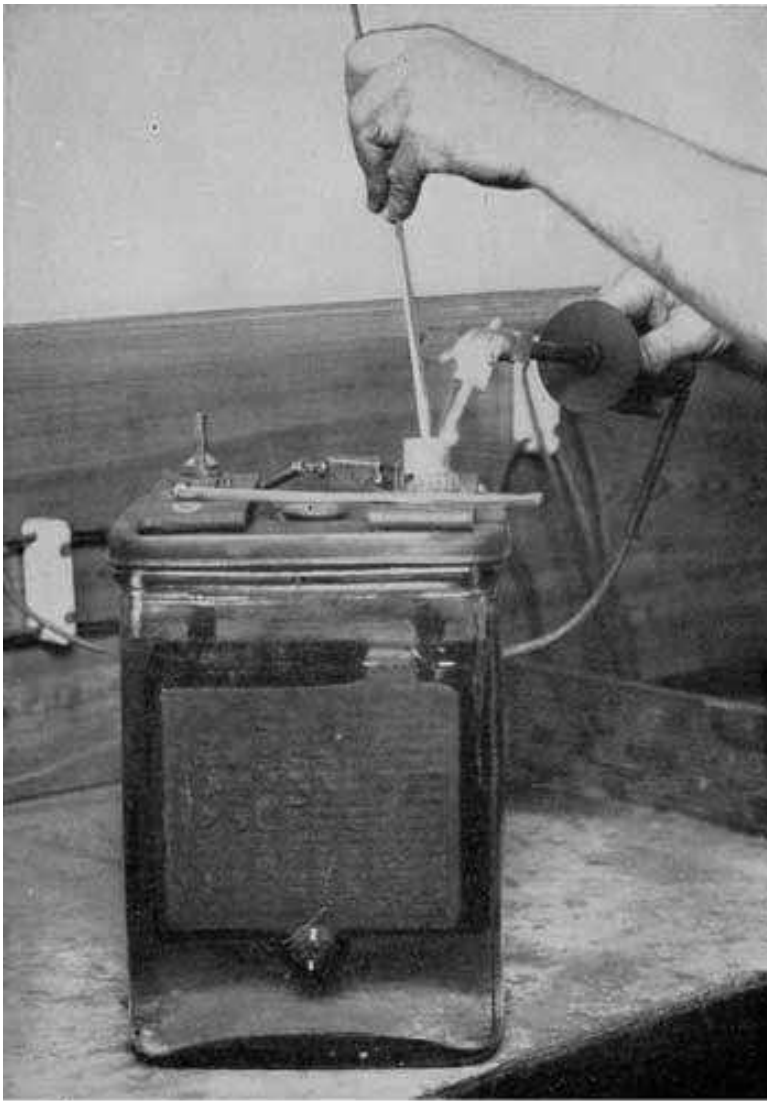
Fig. 319. Burning on Negative Strap. Delco-Light Cell
