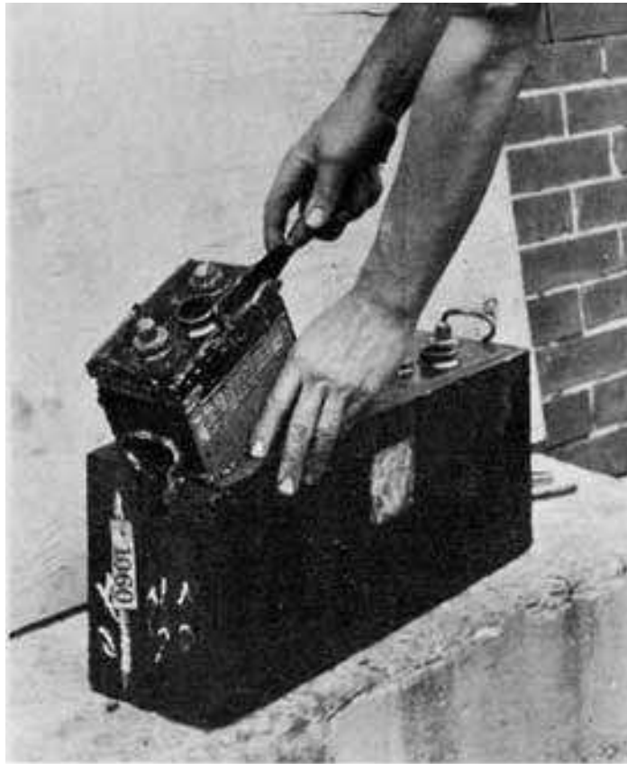
Fig. 198. Removing Compound from Cover
